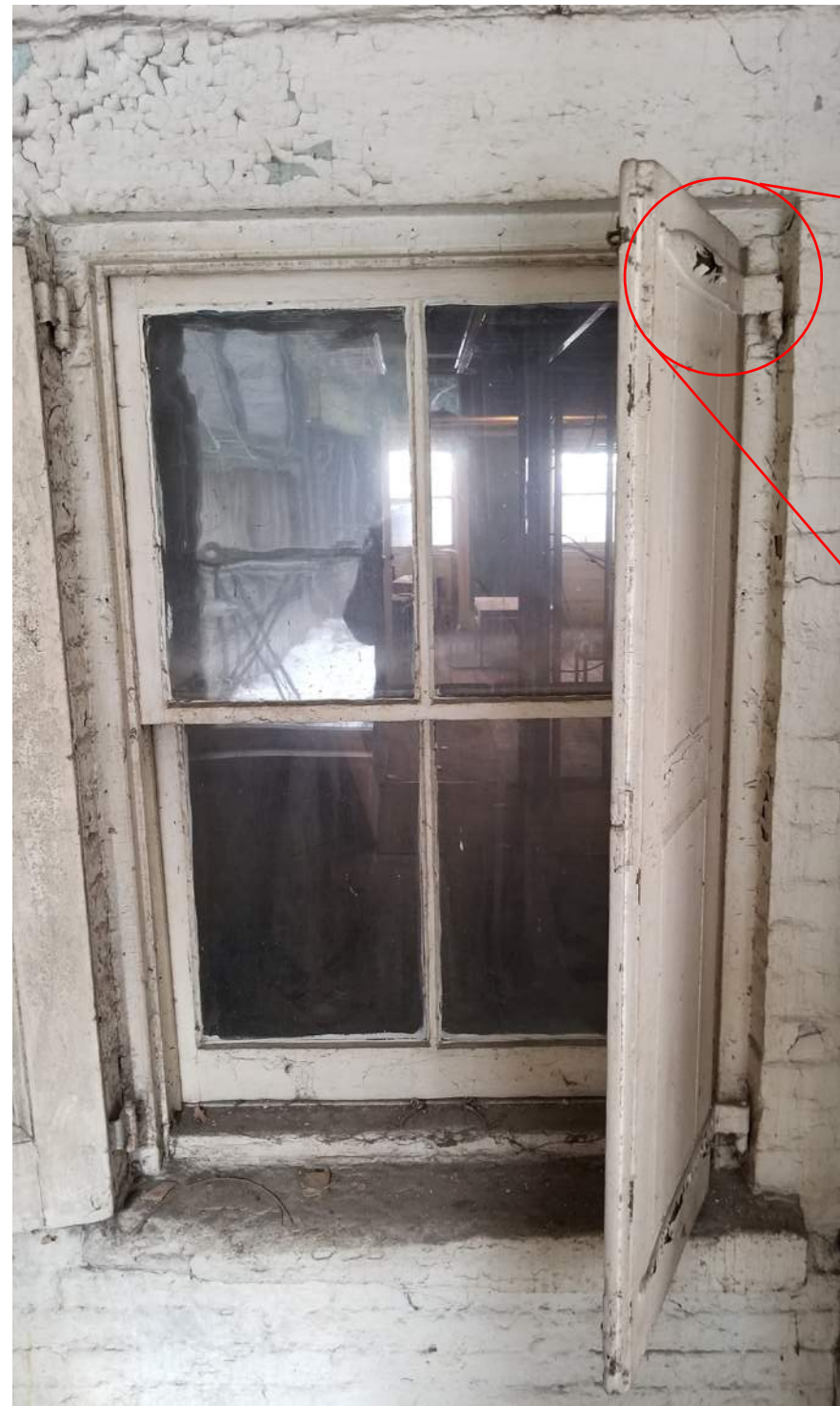
EXISTING SHUTTER HINGE
